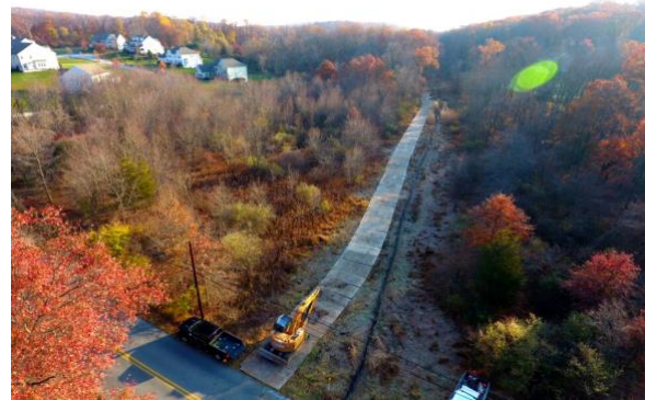
Matting reduces land impact and avoids significant weather delays
