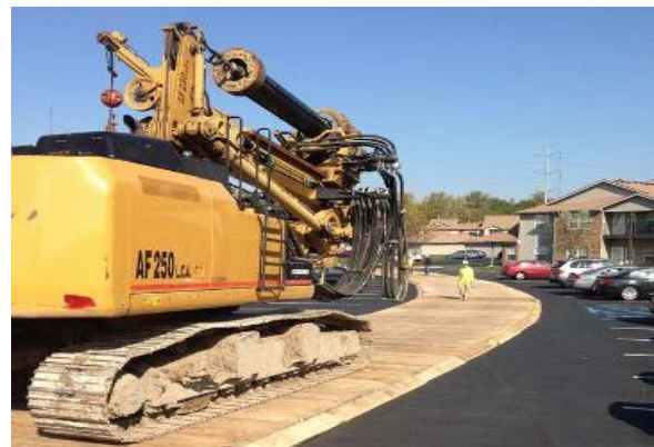
Limited disturbance with Industrial Matting that allows critical access
