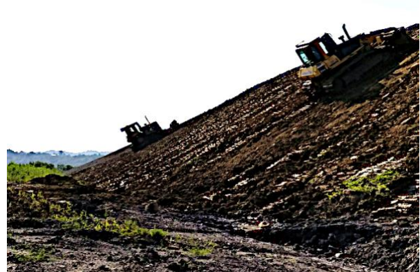
Scarce Topsoil cap incorporated 4"-6" in Lieu of 2 Feet
